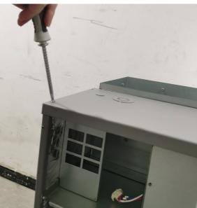
2. Disassemble the electrical box.
