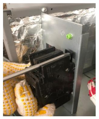
7. Disconnect line voltage from L1 and L2 terminals in control box if applicable. Connect the electric heater molex plug.
