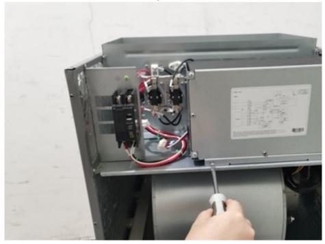
10. Install the front panel and upper panel back to the air handler. Electric heater installation is completed.
